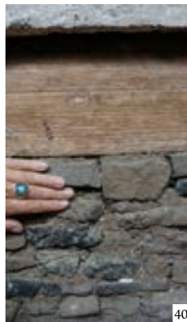
Figure 38: Adjacent building to the church, with wooden structure dissolving in the side wall
