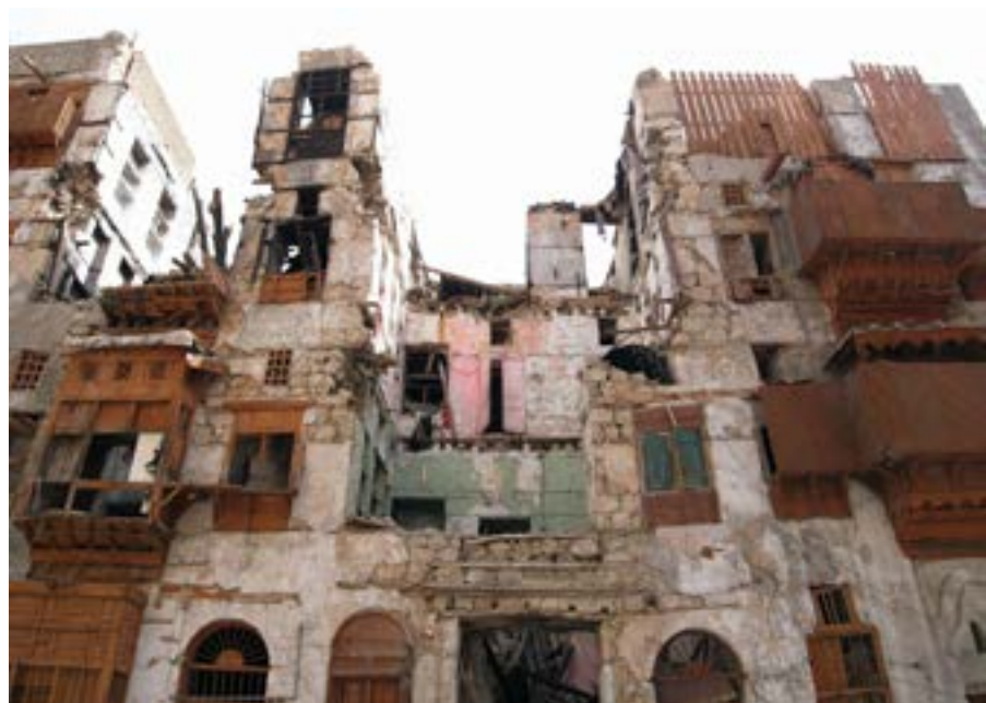
Figure 47: Destroyed building in the old town of Jeddah, which shows the building construction
