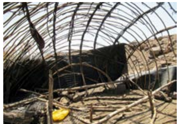
Figure 3: Grid shell made of sticks bound together founded in the ground (Alice Eigner 2011)
