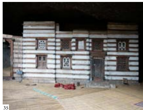
Figure 37: Yemrehana Kristos church in the Lalibela region, mid-12th century, with classical features of Axumite architecture: horizontal layering of masonry and wood, rows of windows and edge parts of the building projecting out
