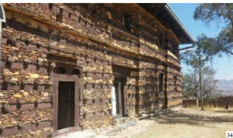
Figure 37: Yemrehana Kristos church in the Lalibela region, mid-12th century, with classical features of Axumite architecture: horizontal layering of masonry and wood, rows of windows and edge parts of the building projecting out
