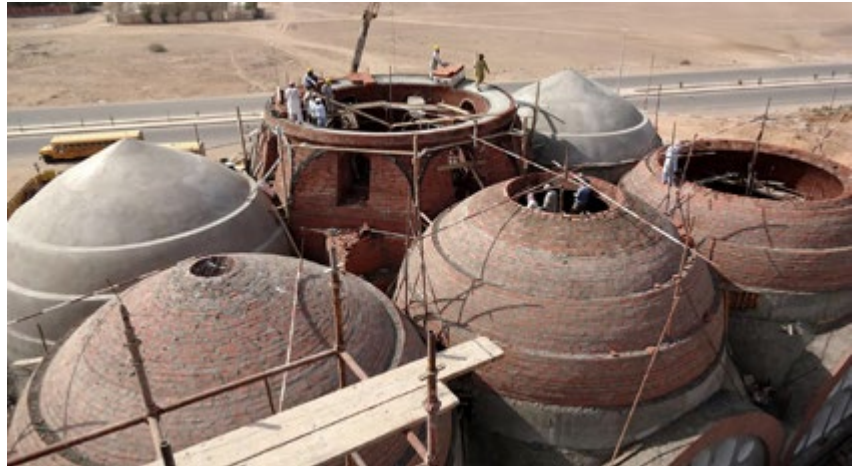
Construction of the six domes over the main hall | Construcción de las seis cúpulas sobre la sala principal | Construção das seis cúpulas sobre a sala principal (Ghazi El-Maimani group)
