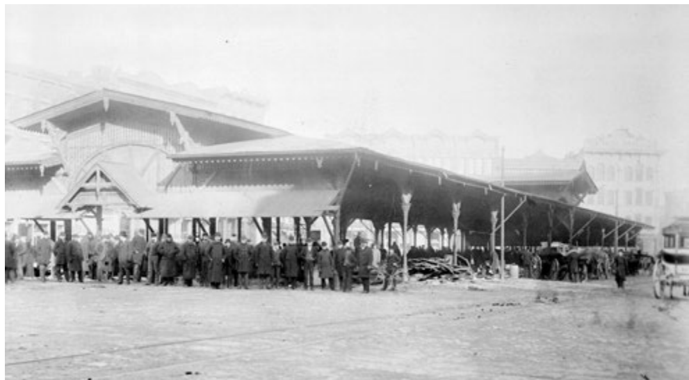
Figure 2. The timber frame market building being deconstructed in 1892 under police guard (From the collections of The Henry Ford)
