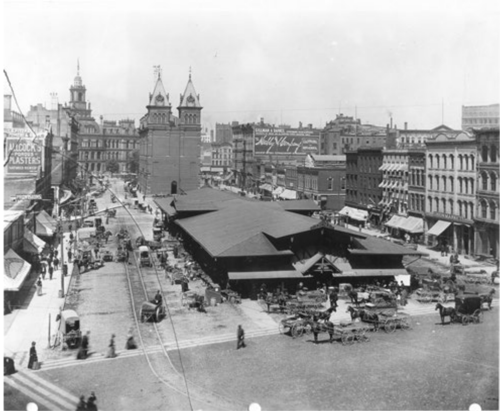
Figure 1. The Detroit Central Farmers Market with the timber-framed vegetable shed in the foreground and the masonry meat market in the background, c. 1880 (From the collections of The Henry Ford)
