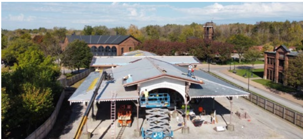
Figure 23. Drone view of the building and surrounding area as slate roofing began (From the collections of The Henry Ford)
