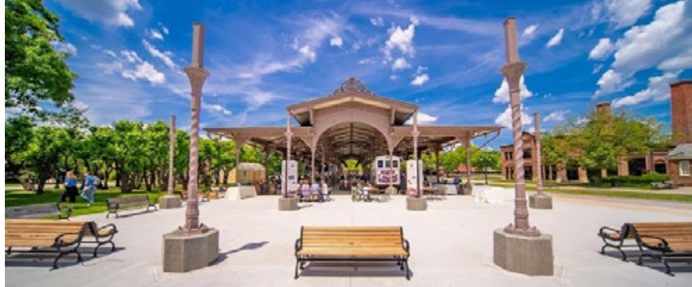
Figure 24. Completed market building with added rows of salvaged cast-iron columns to give visitors a sense of its original size (From the collections of The Henry Ford)
