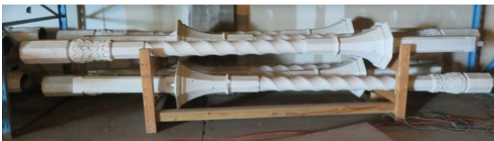
Figure 7. The original cast-iron columns were cleaned, prime-coated and put into storage (Christian & Son, Inc.)
