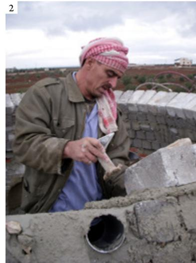
1: Construction of vaulted ceilings using composite blocks. Dar Al-Shiek - Horan, Syria
