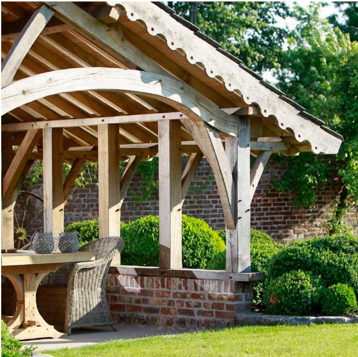
Timber shade structure built by Mortier in his own garden
