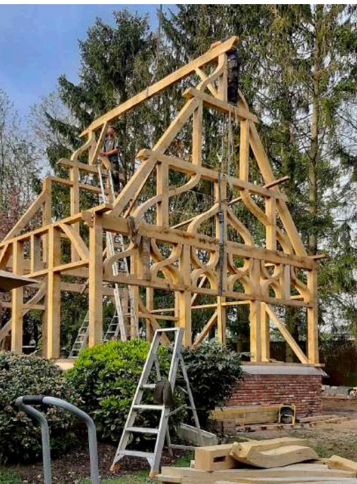
Eclectic half-timber residence in Koersel, completed in 2018
