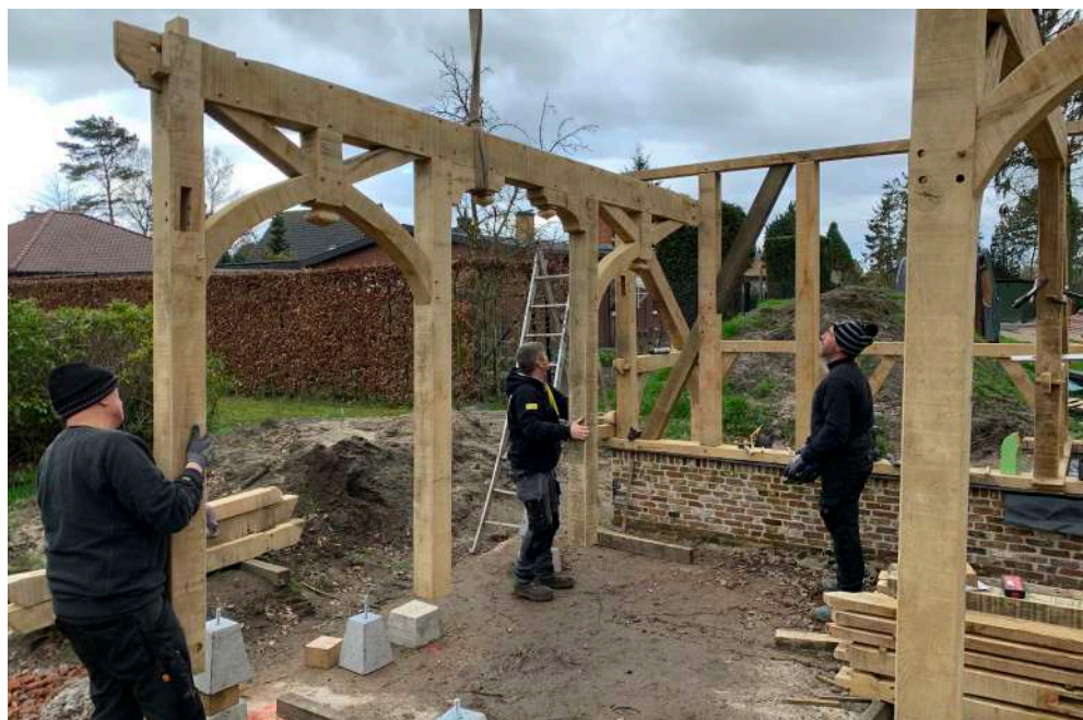
Installing the timber framework on site
