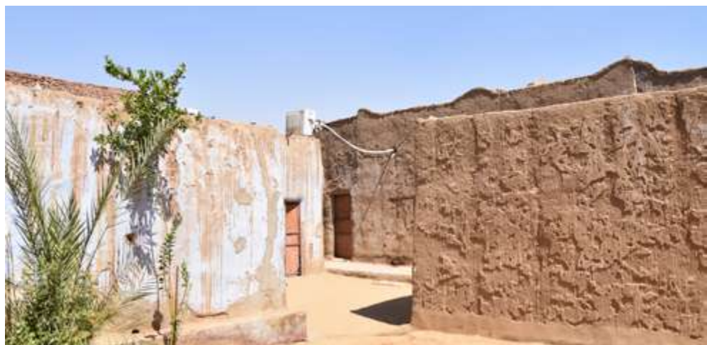
View from the huash to private domestic spaces
