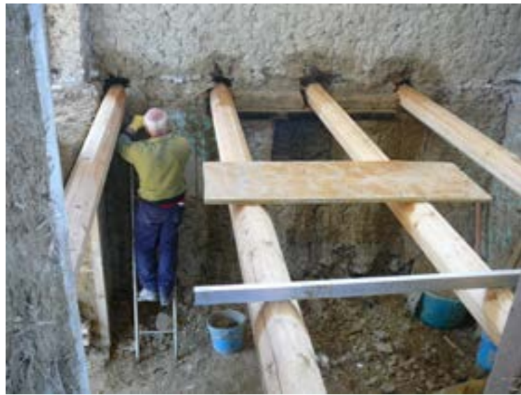
Figure 24: Laying the new beams in the west room (CEDTerra)
