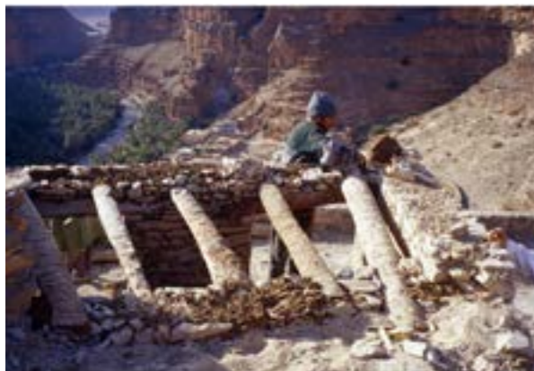
Agadir n'Uguellouy, Western Anti-Atlas, restoration works in progress
