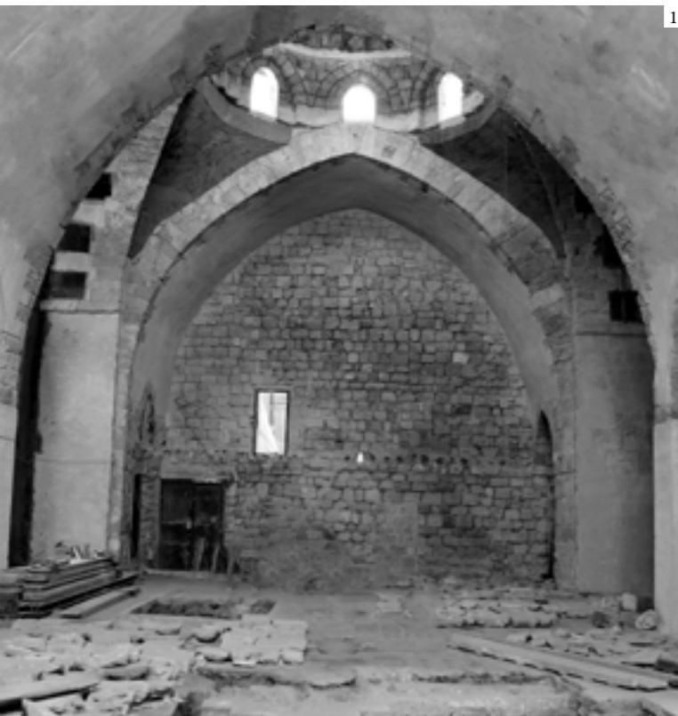
Condition of the interior before restoration (1) and Interior view looking towards the new mezzanine (2) of the Masjid Al Attar, Tripoli, Lebanon, 2019 - In progress
