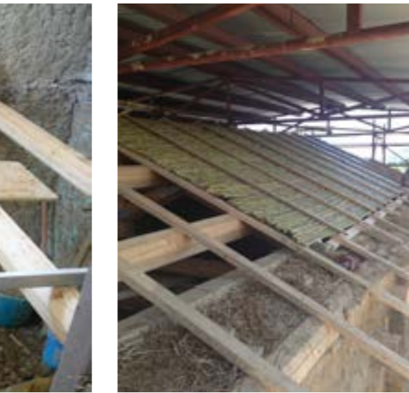
Figure 25: Laying of the laths made during the 2015 workshop (CEDTerra)
