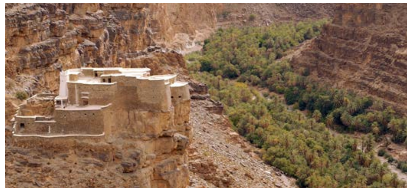
Agadir n'Uguellouy, Western Anti-Atlas, just after the restoration of 2016, photograph by drone (M. Benssid)
