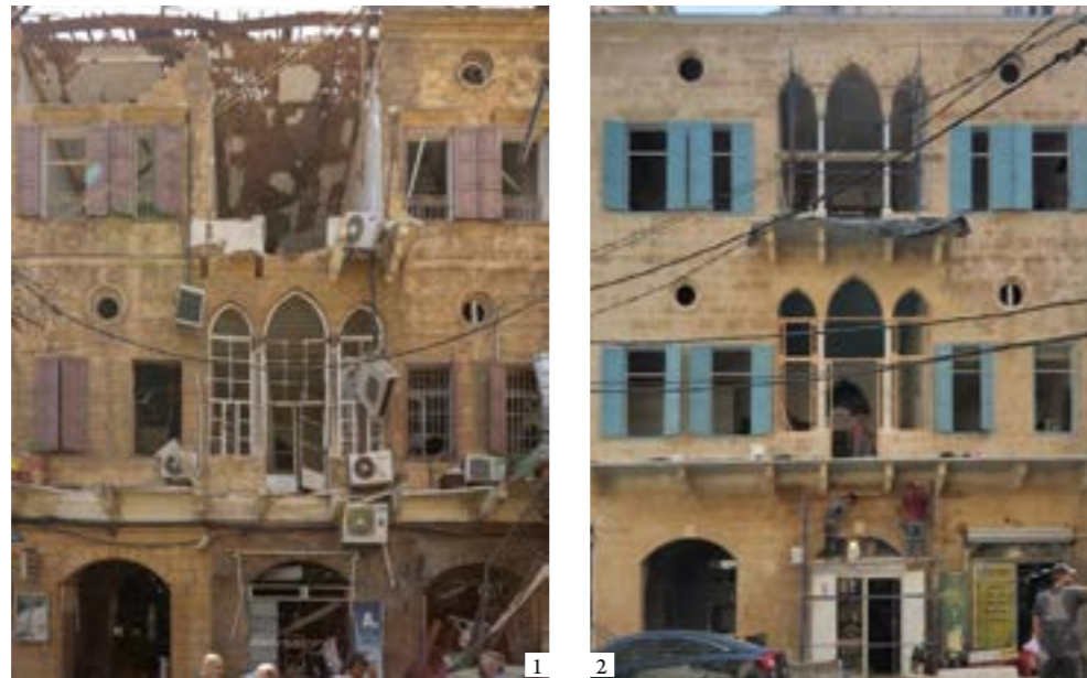
1: Rmeil 722 north facade after the blast (Dia Mrad) 2: Rmeil 722 north facade after restoration
