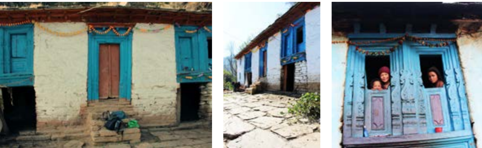
Figure 17. Photographs showing the facade and window details
