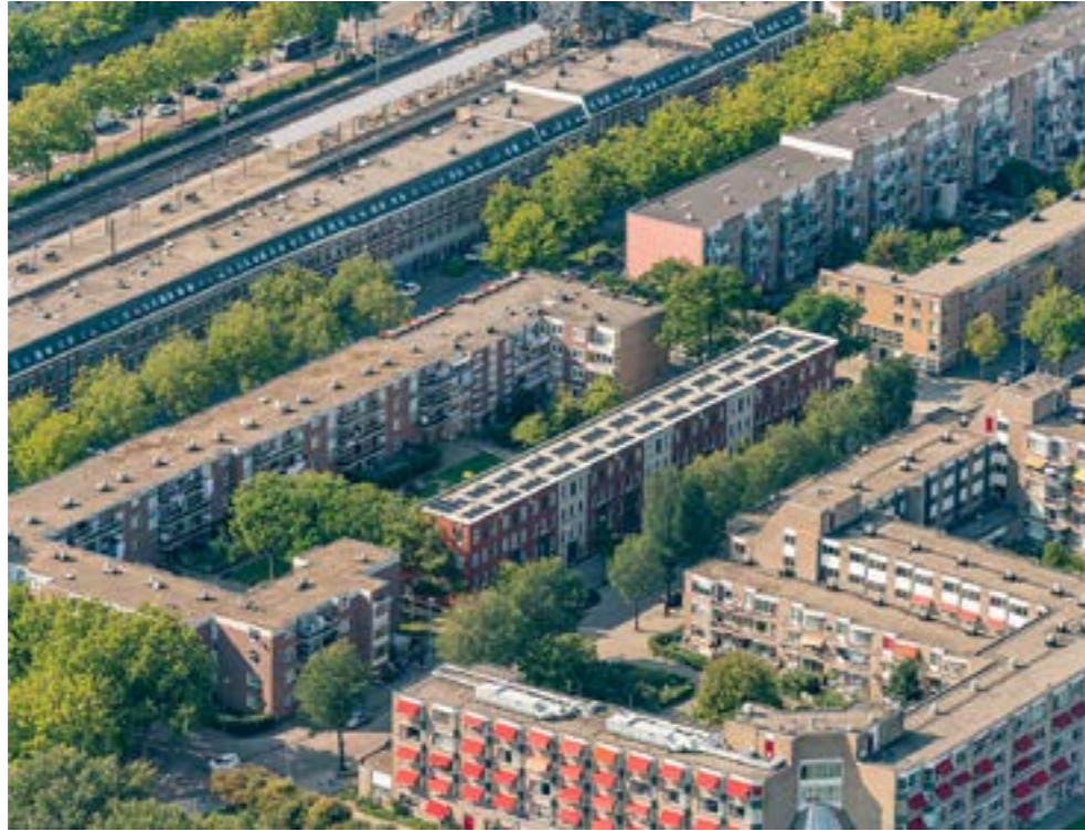
Aerial view of the project site
