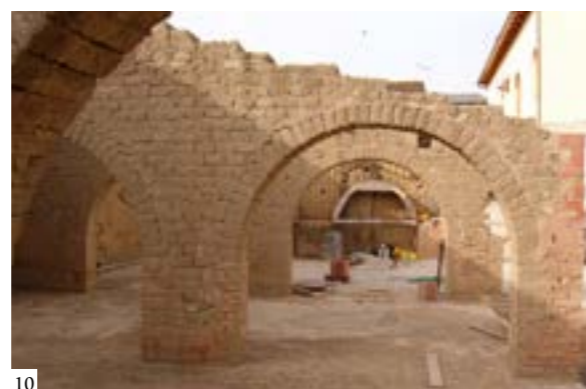
Figure 7: In the reconstruction work of building B, the reuse of original ladiri in good condition was frequent. The earth derived from the demolition, heterogeneous and with spurious materials, was not reused within the construction site, but was instead reused to fill the land where the earth used for the new bricks was extracted from. (Ignazio Garau)
