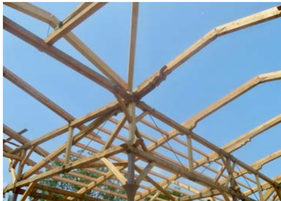
Figure 9. View of the finished frame showing the added compression post/tension rod system installed (Christian & Son, Inc.)
