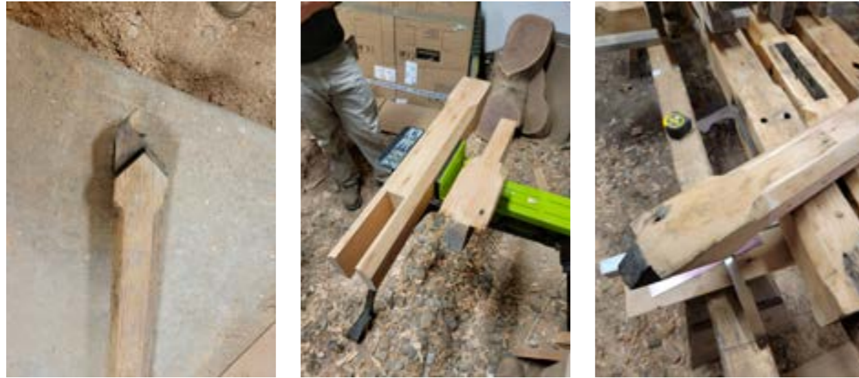
Figures 15, 16 and 17. Brace tenons damaged during installation of the added monitor trusses required blade-and-fork repairs with salvaged ends from damaged braces (Christian & Son, Inc.)
