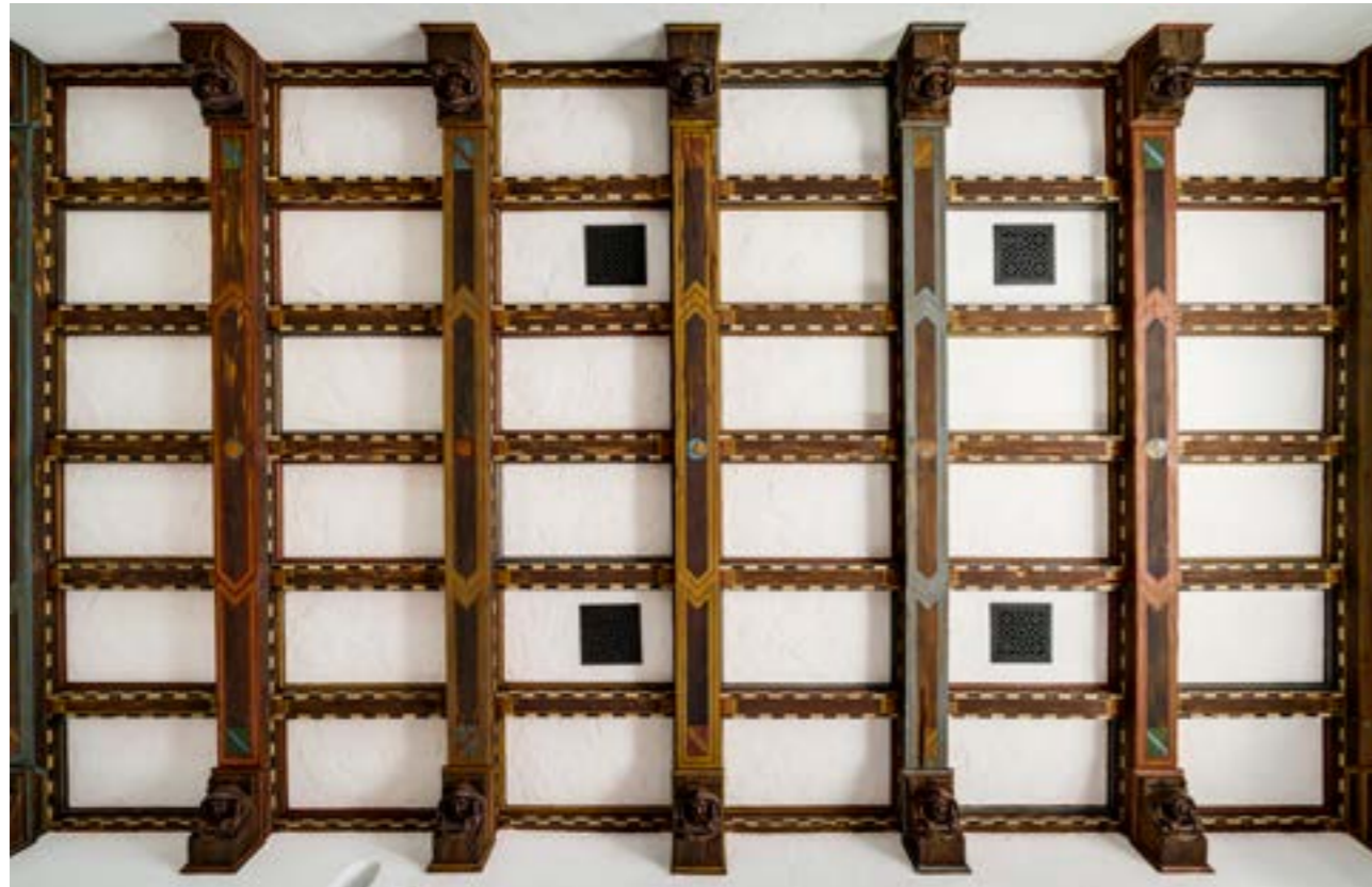
Restored ceiling | Techo restaurado | Teto restaurado (Alex Tarajano)
