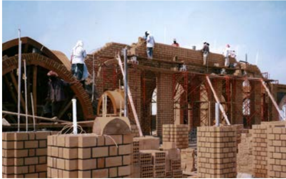
Construction of Dar Al Qasir, Manama, Bahrain, 1995
