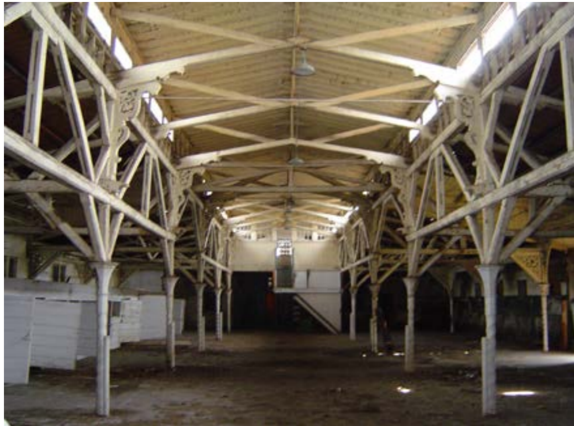
Figure 5. The interior of the Riding Academy building revealed a very well-built and highly decorated timber frame plus the added monitor and support framing (Christian & Son, Inc.)
