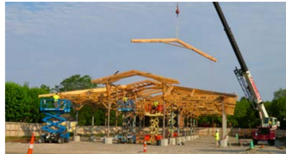
Figure 22. As the historic roof frame sat on top of 15-foot cast-iron and steel columns, installation had to be done with manlifts, extendable forklifts and a crane (Christian & Son, Inc.)
