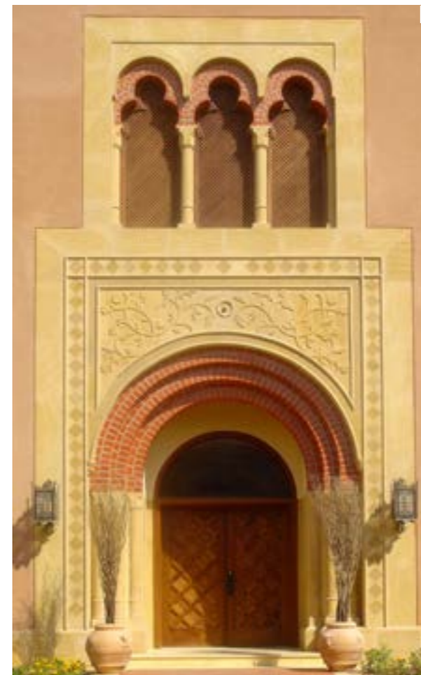
1: View looking towards the wooden mashrabiya of Dar Al Fahim 2: Detail of the interior ribbed vaults in the ground floor gallery 3: View of the carved stone and brick entrance portal
