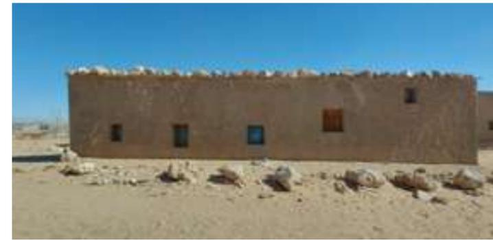
Figure 16: Facade of a housing unit in the *wilāyah* of Smara. Openings at different heights, reflecting the use of interiors and facilitating cross-ventilation (2022)
