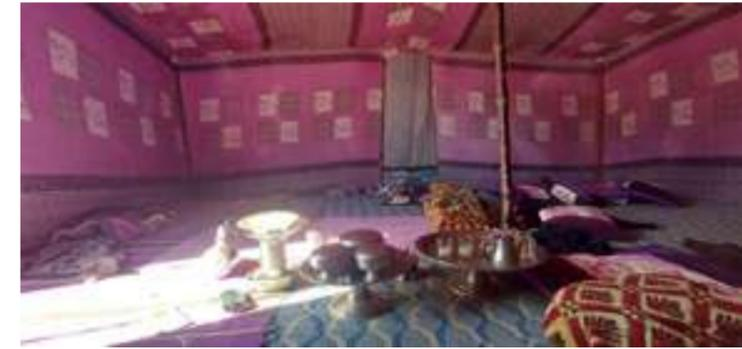
Figure 17: Interior of a tent in the *dā'ira* of Dcheira, *wilāyah* of El Aaiún. The tent structure consists of metal poles in the sides and two bamboo posts about 4 m high. There are four layers of textiles: a strong dark cotton fabric as the exterior, a second layer of light cotton, a third one of old fabrics such as veils and rags, and finally the fabrics of the interior furnishings. These layers along with the tent's shape and orientation make it comfortable even in the hottest hours
