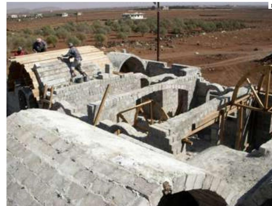
1: Construction of vaulted ceilings using composite blocks. Dar Al-Shiek - Horan, Syria
