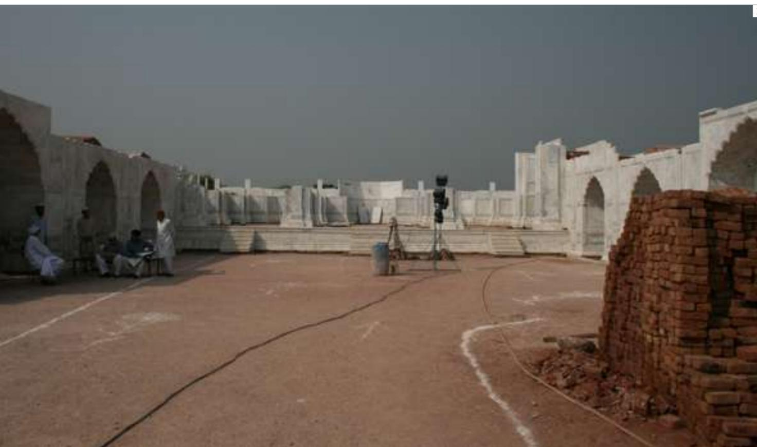
had set, the foundations were built to a height of 12 feet above ground in order to create what is known locally as a *takht*, or bed, on which the mosque was to be erected. At no point during the process was any steel or concrete used and a strict adherence to traditional building materials was observed. While at times this approach did lead to a considerable increase in cost, it was felt that the use of modern materials would pollute the site, compromising its sanctity.
