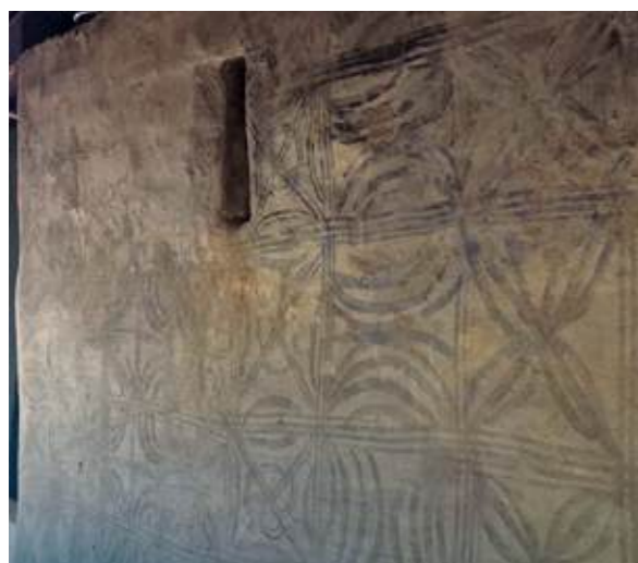
Figure 24: Earthen dwelling with mud plaster (Wayanad, India, 2018)
