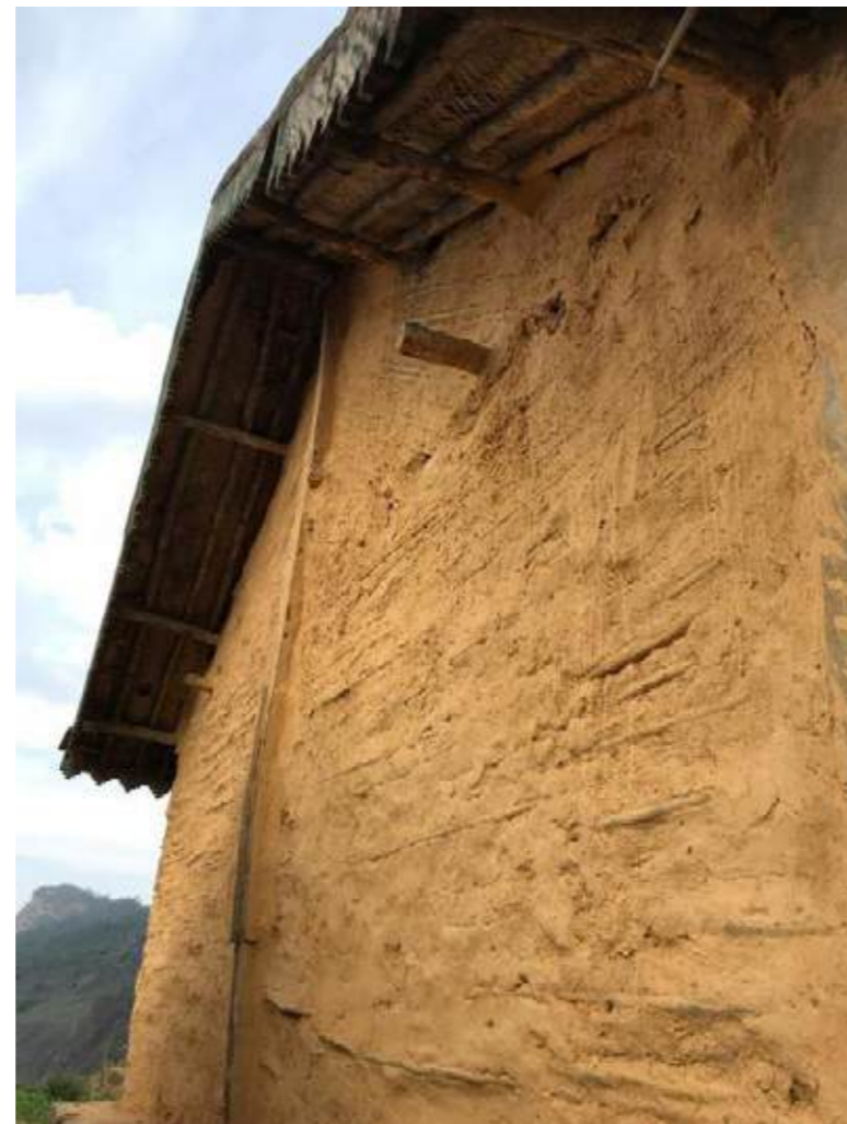
Figure 1: Traditional wattle and daub dwelling with earthen plaster (Kookal, Tamil Nadu, India, 2019)
