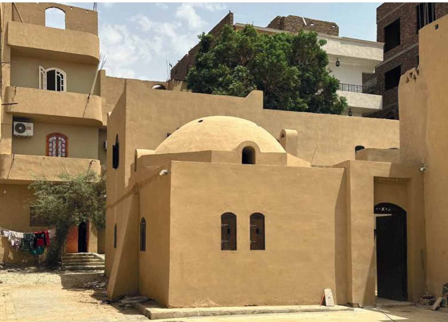
Figure 20: Fathy's house, before and after restoration | Casa de Fathy, antes y después de la restauración | Casa de Fathy, antes e depois do restauro
