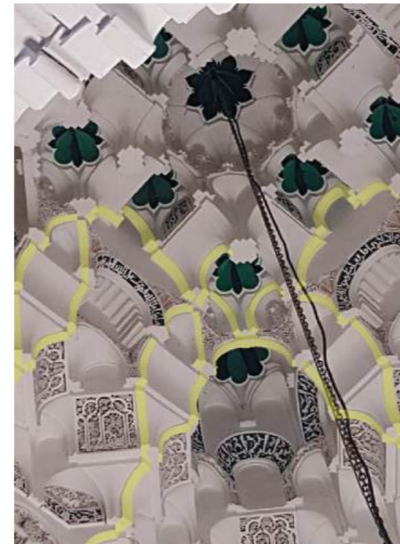
Figure 8. The ktib element in muqarnas at the Qarawiyyin Mosque, Morocco (highlighted in yellow)
