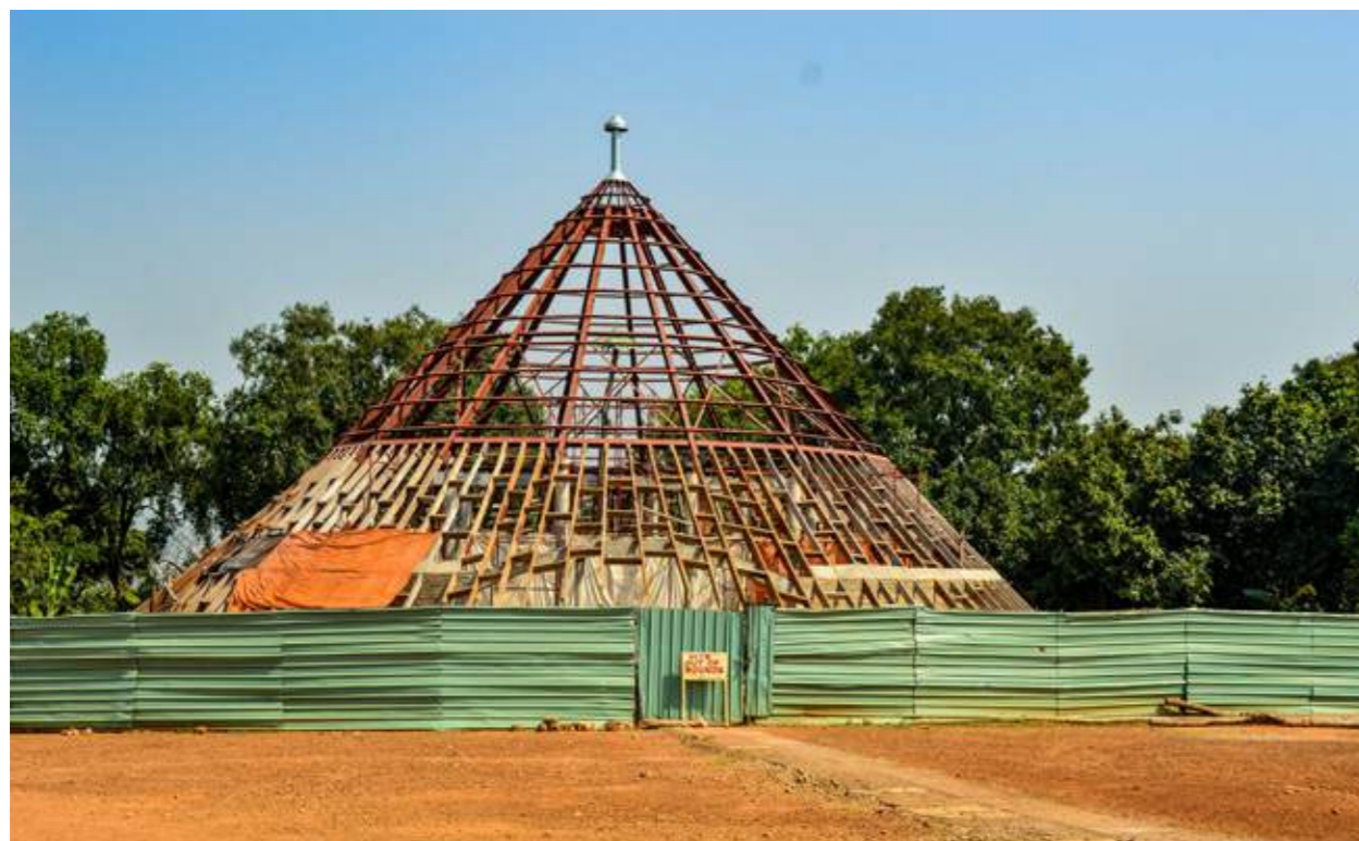
Figure 18: Kasubi tombs building being rebuilt after burning down (Alamy)
