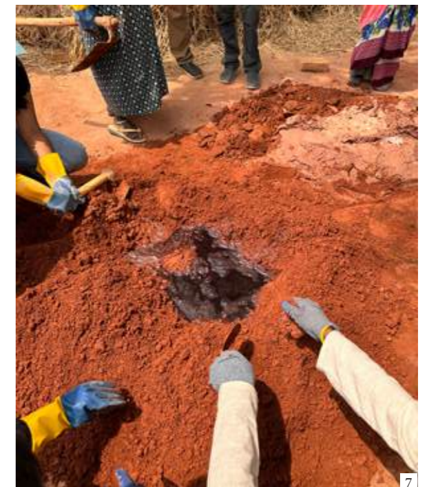
Figure 7: Addition of jaggery and fenugreek water (Bagalur, India, 2023)
