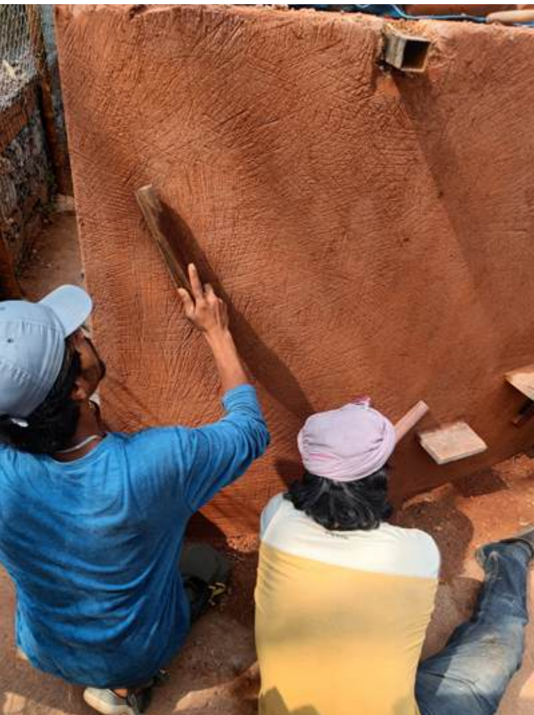
Figure 3: Thappi plastering with the eponymous wooden tool (Bagalur, India, 2023)
