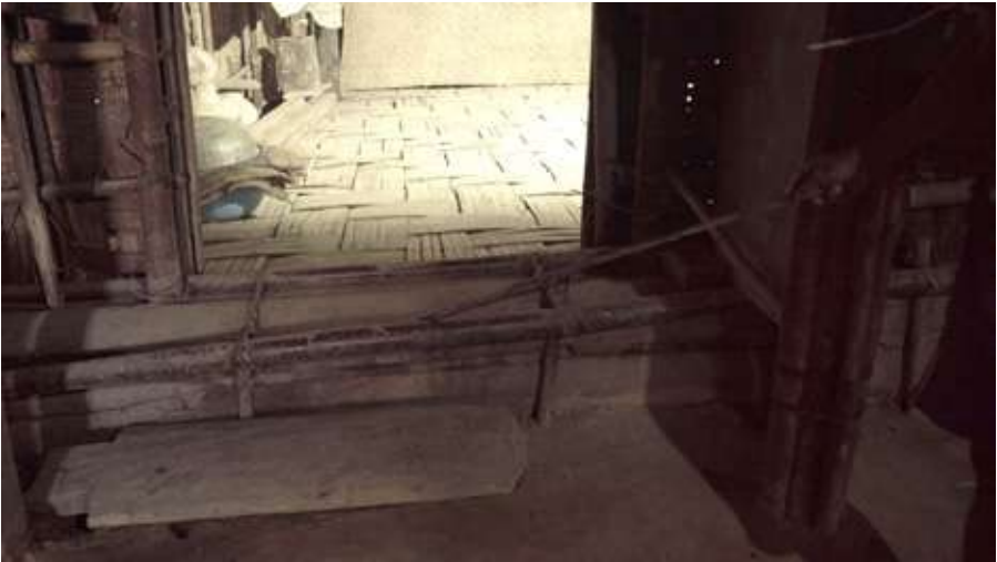
Wapan base beam dividing the phongkha from the kamkey (back room) in Hondan Losu’s house, Kamhua Noknu, 2023
