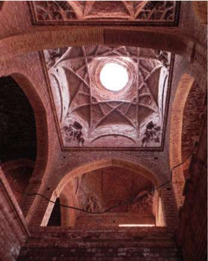
Ribbed dome | Cúpula nervada | Cúpula nervurada
