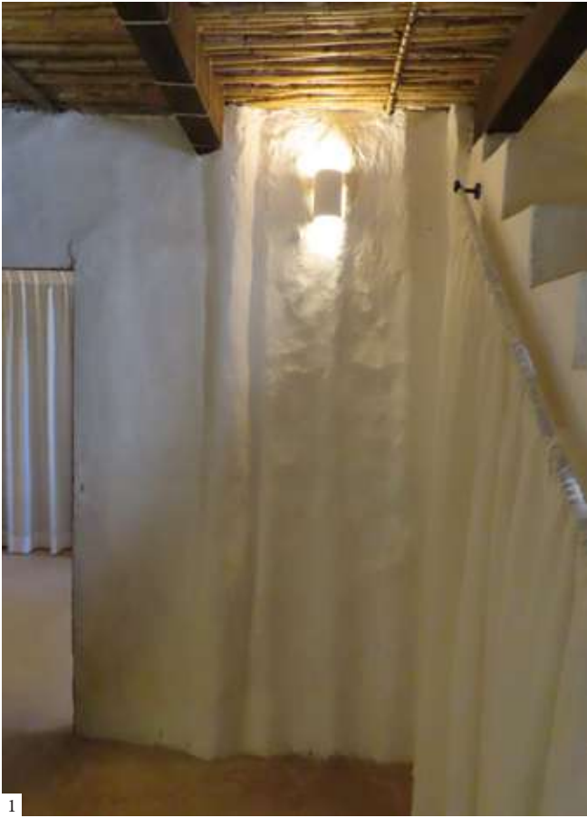
1: Detail of the restored reed partition wall, plastered with clay and whitewashed with lime, dating from the 18th century 2: Interior of the cottage after restoration | 1: Detalle de la tabiquería restaurada de encañizado enlucida de barro y encalada de cal que data del siglo XVIII 2: Interior de la barraca después de la restauración | 1: Detalhe da divisória restaurada de caniço, rebocada com barro e caiada com cal, datada do século XVIII 2: Interior da cabana depois da restauração
