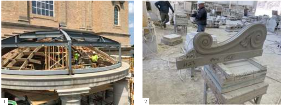
1. Erection of the portico dome shoring at Christ Chapel 2. Carved limestone bracket in progress for the front entrance at Christ Chapel
