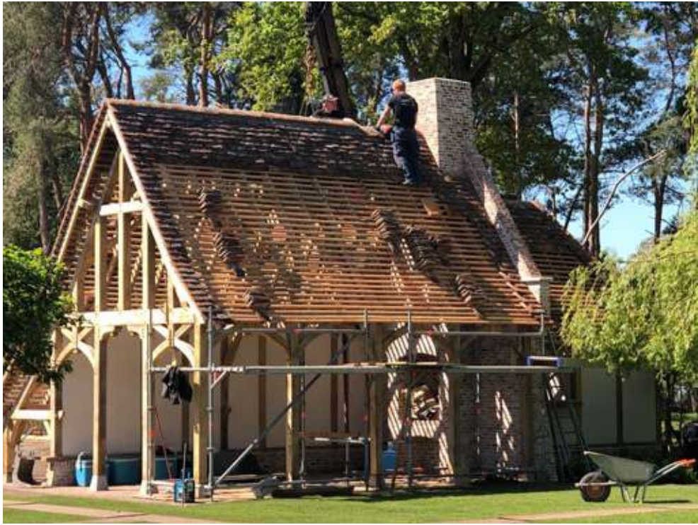
Roofing work underway on the De Wilde–De Scheppe project
