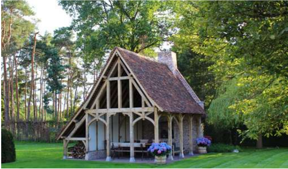
Completed timber pavilion
