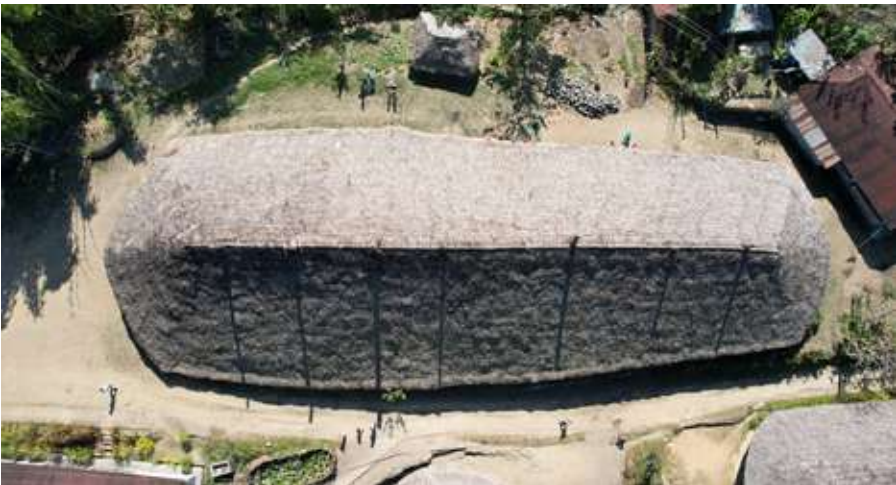
Drone view of the wangkam roof, Kamhua Noknu, 2023 (Angam Wangpan)
