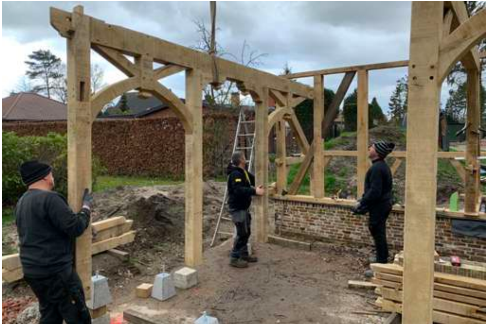
Installing the timber framework on site
