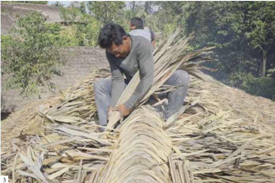
1. Detail of door and woven bamboo walls (Arnav & Anupama Architects) 2. Completing the reconstruction of the wangkam (chief’s house) in Kamhua Noknu in 2021 3. Ogeeko process of wrapping the central ridge pole (ochung), Kamhua Noknu, 2023
