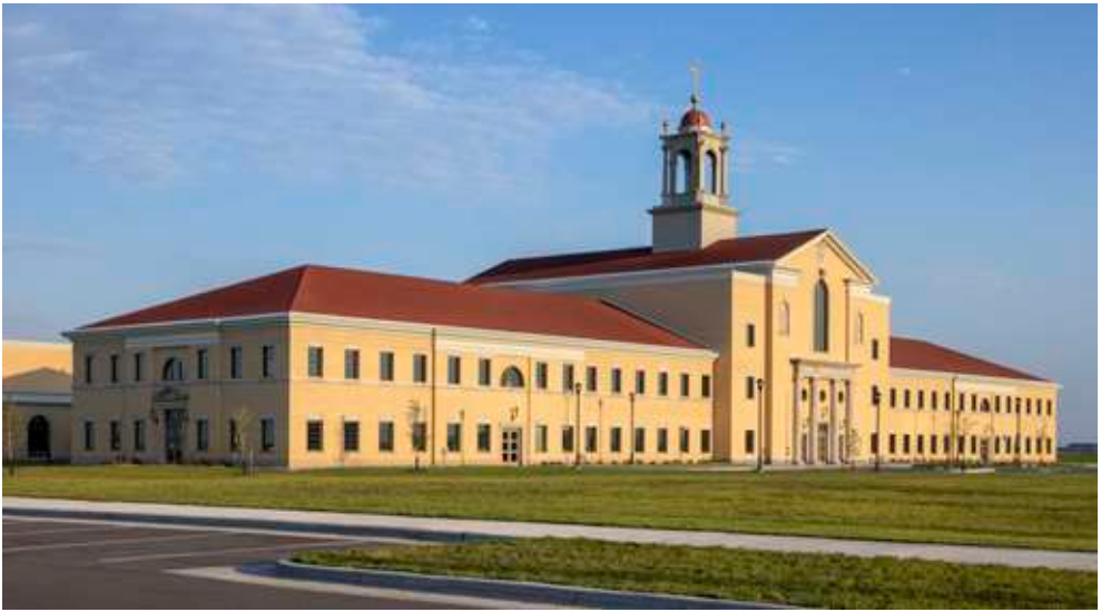
Capstone Classical Academy, completed in 2025 (Francis Dzikowski/Otto)
