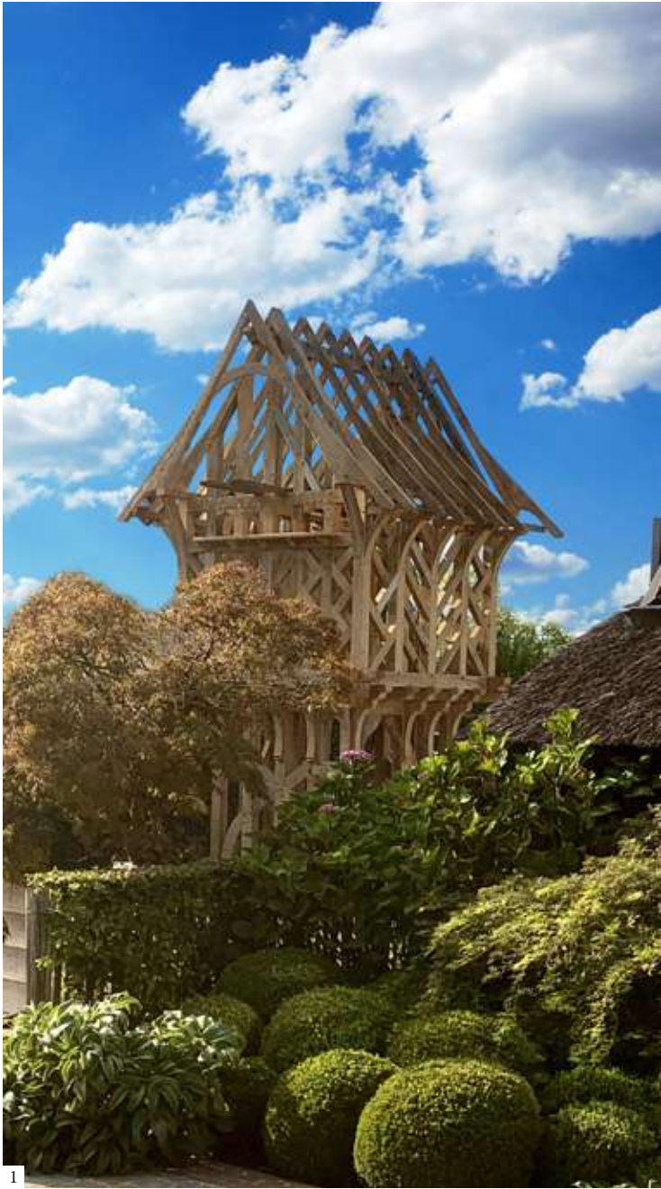
1: Timber-framed pigeon tower built for a landscape exhibition in Beveren-Waas, Belgium
