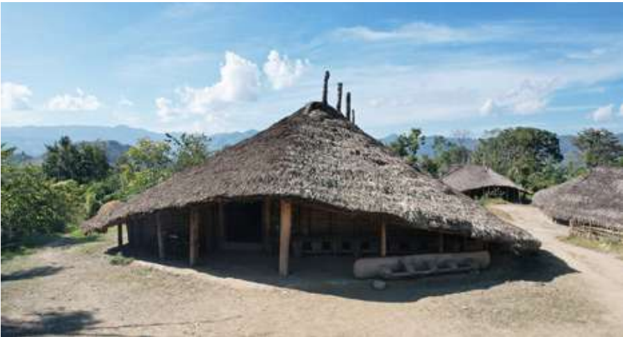
Drone view of front of the wangkam in Kamhua Noknu, 2023 (Angam Wangpan)
