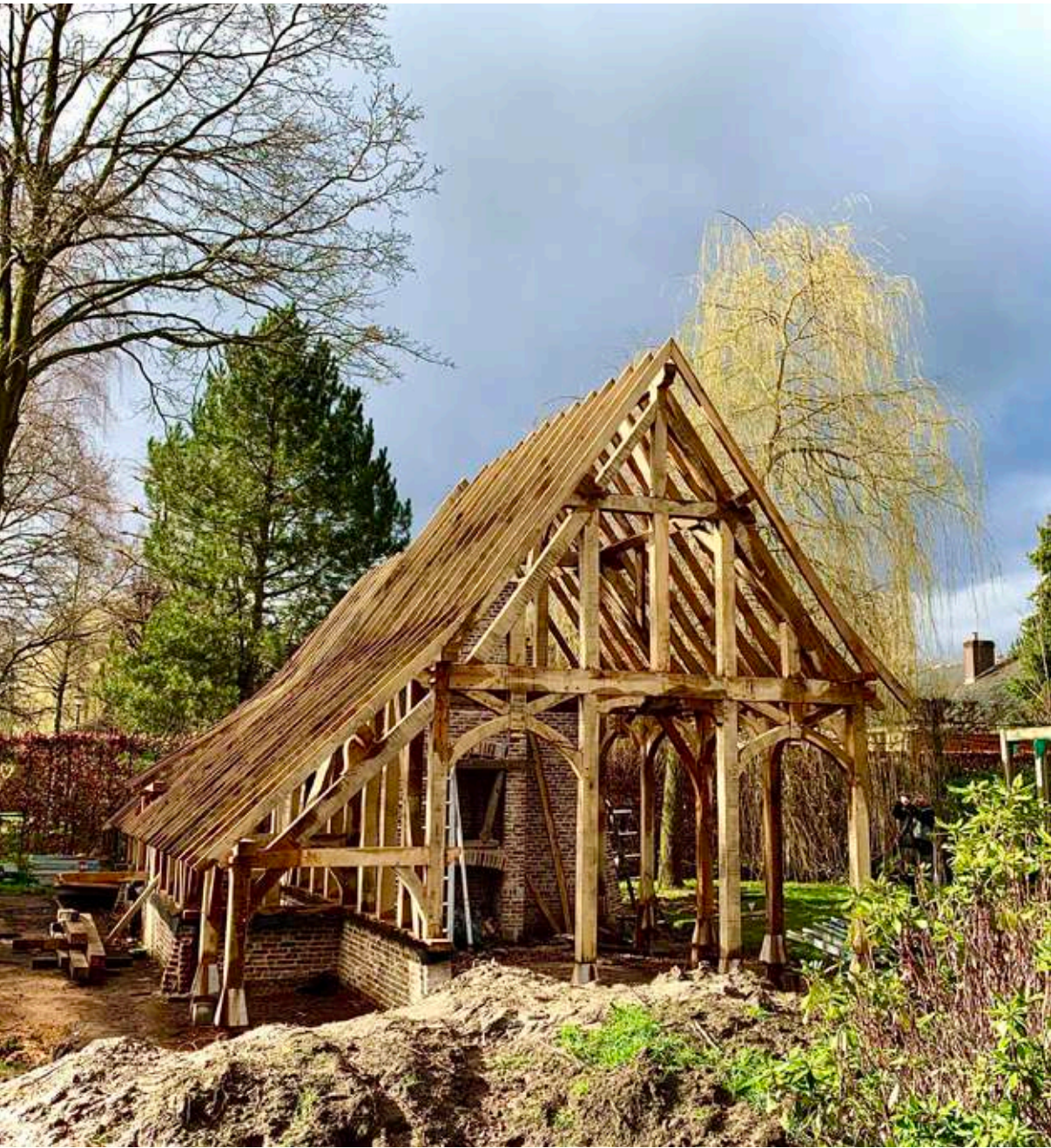
Assembled timber truss during the erection of the structure in Laarne
